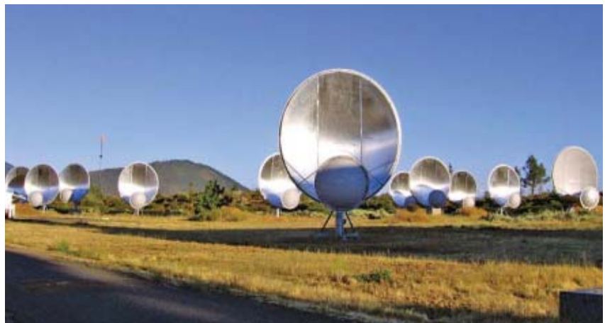
[FIG1] The ATA, activated in October 2007, is a joint project of UC-Berkeley and the SETI Institute. Currently made up of 42 radio dishes, the system is expected to grow to 350 dishes to advance the search for extraterrestrial life and radio astronomy research.
